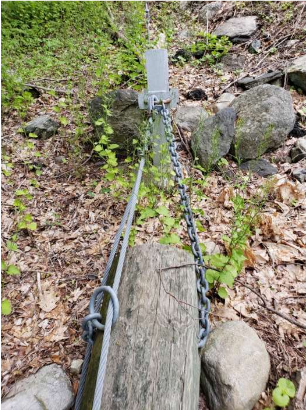
Informational Photo 3 – East anchor- cable will remain and chain to be replaced.
